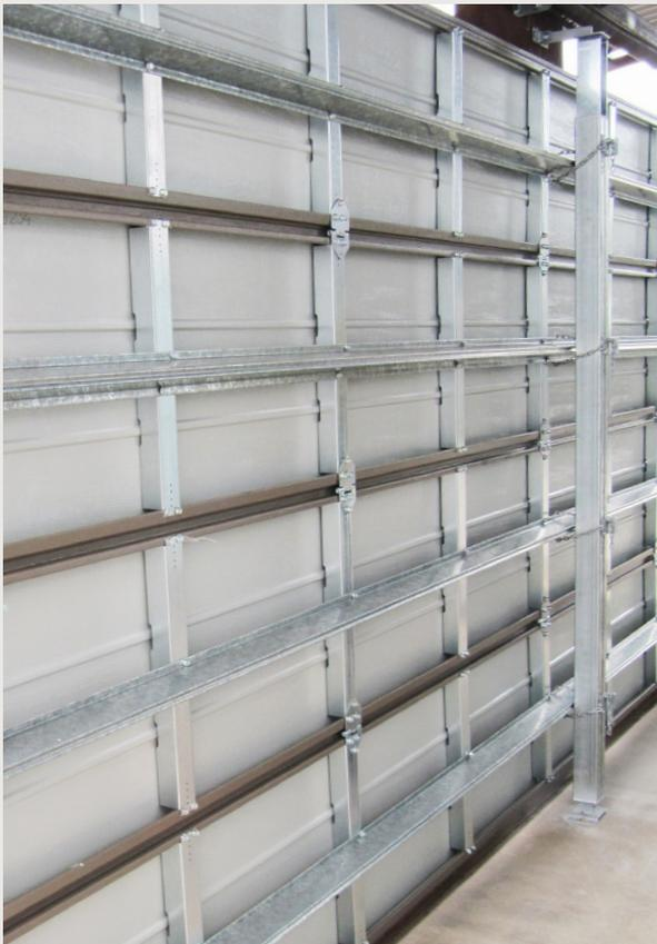
Typical Post to Strut Connection Details
